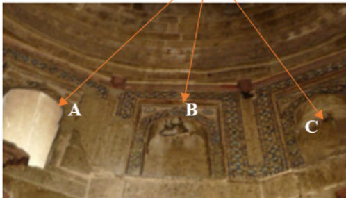
Sixteen sided drum at the top of octagonal base
